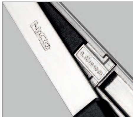
ABOVE: A simple mechanism releases the window in the event of fire to provide a safe exit.
